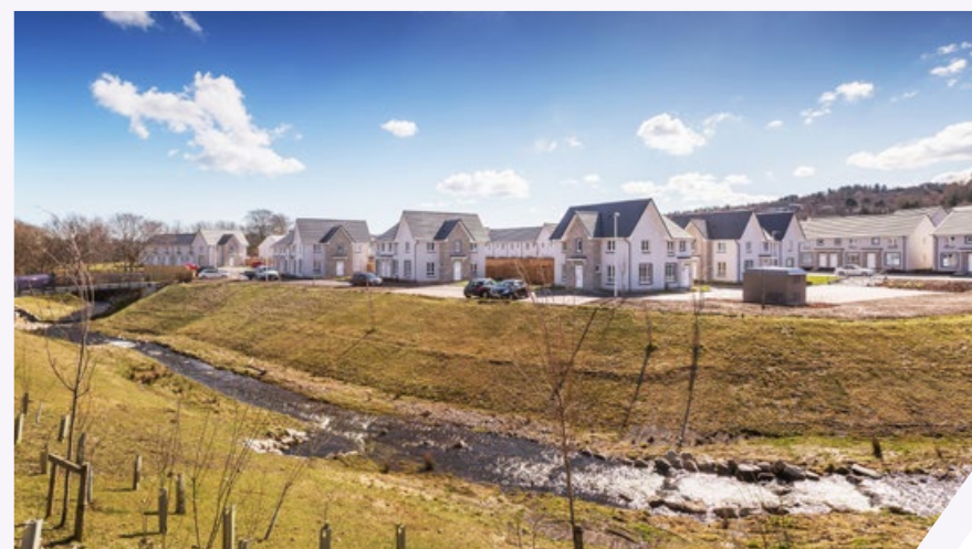
Views across the development and the 'daylighted' Bucks Burn which now provides a focus for the development and greater wildlife opportunities.
