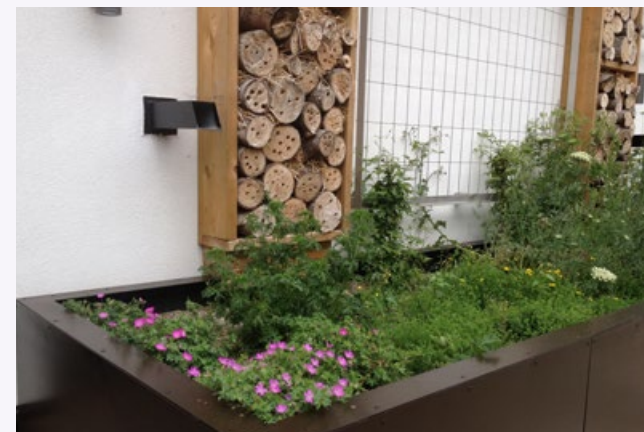
Figure 14 Conventional and raised planter rain gardens served by water from a downpipe
