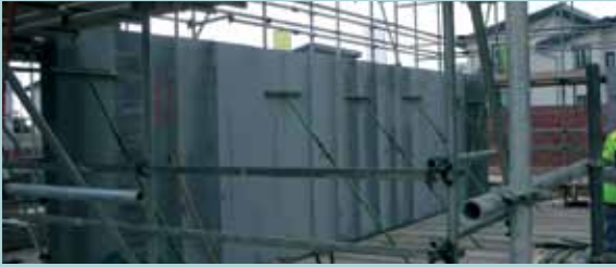
The Code Level 6 aircrete panel house under construction
