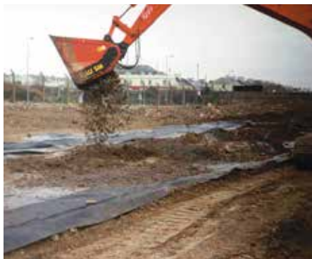
Figure 6.8 Bio-remediation of soils (ex situ)
