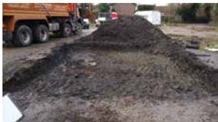
Figure 6.5 Excavation and disposal
