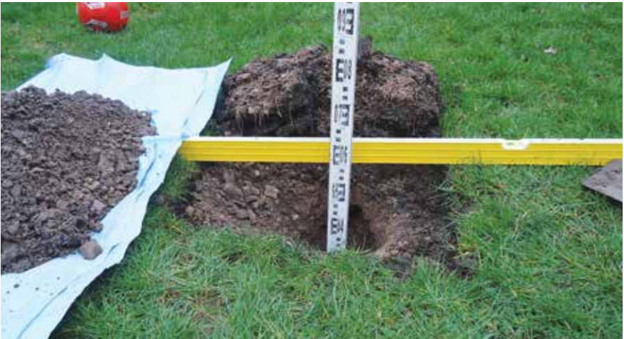
Figure 6.9 Verifying the depth of a clean cover system
