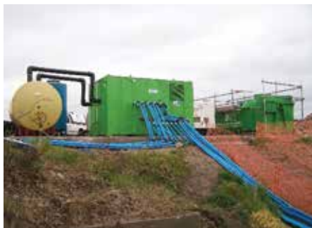
Figure 6.6 In situ soil and groundwater remediation
