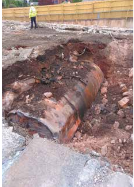
Figure 8.2 Work in progress to remove a disused underground tank (courtesy Curtins)
