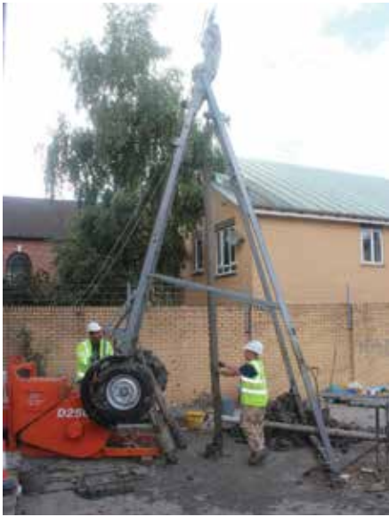
Shell and auger drilling
