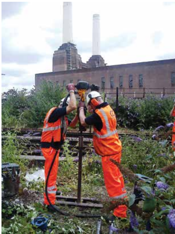
Figure 5.5 Hand-held portable drilling equipment
