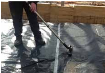
Figure 6.4 Ground gas protection systems
