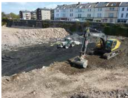
Figure 6.7 Soil solidification and stabilisation
