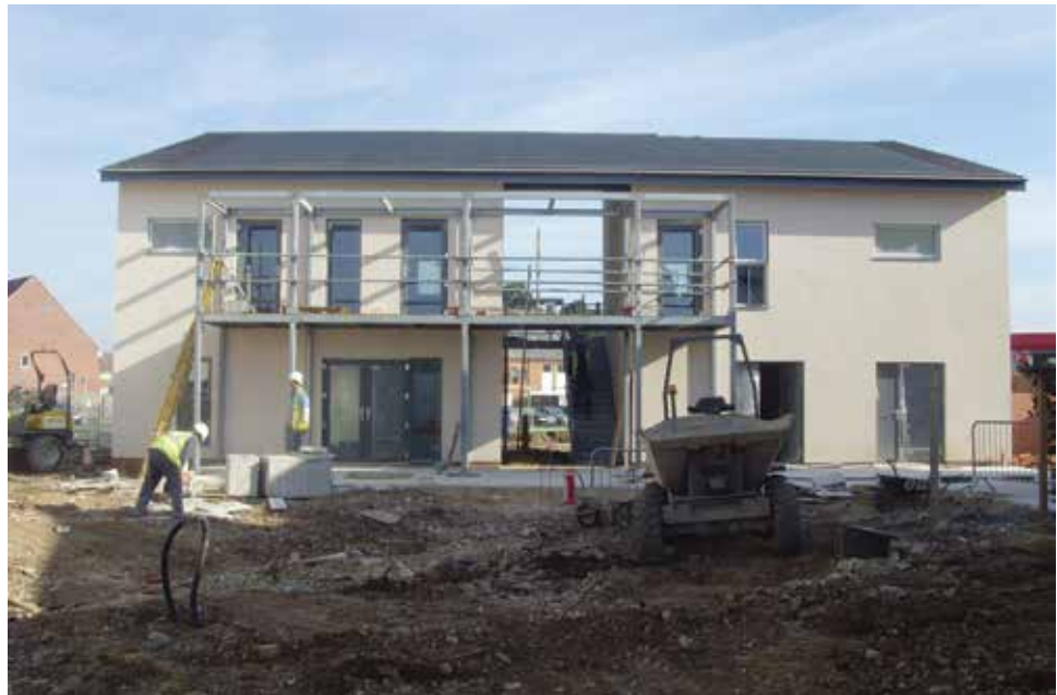
Figure 4 Greenwatt Way (Homes 5 and 6) shown during construction
