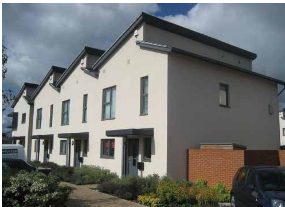
Figure 3 Greenwatt Way in Chalvey, near Slough, Berkshire
