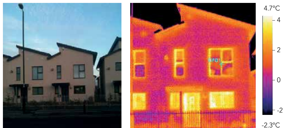
Figure 7 Front façade of Home 2. Corresponding thermal image shows uniform heat loss across the building façade
