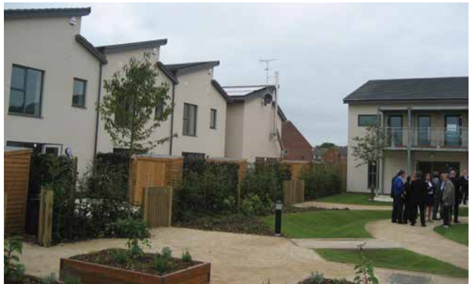
Figure 5 Homes 2 to 4 (left), energy centre (middle) and Home 5 (right) shown on opening day
