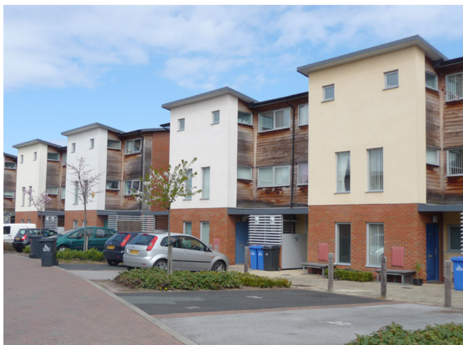
Figure 14 Waterbridge Mews, the first phase of the Castlefields Estate Regeneration Project to trial the closed panel timber frame system
