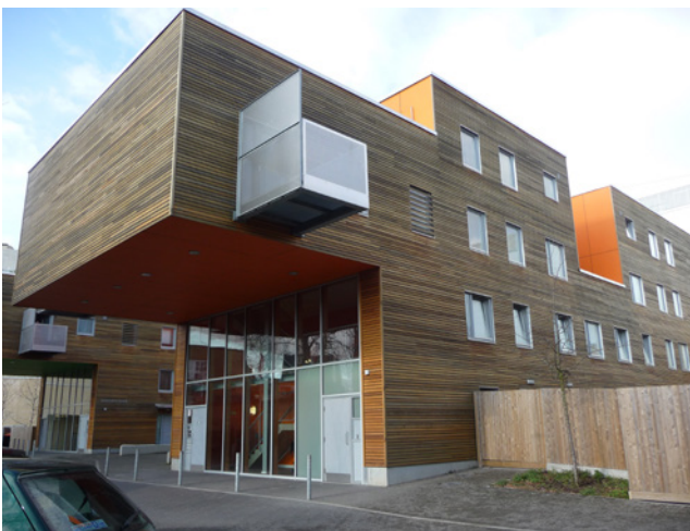
Figure 19 The steel frame was designed to allow the upper floors to cantilever over the access road, increasing plot density
