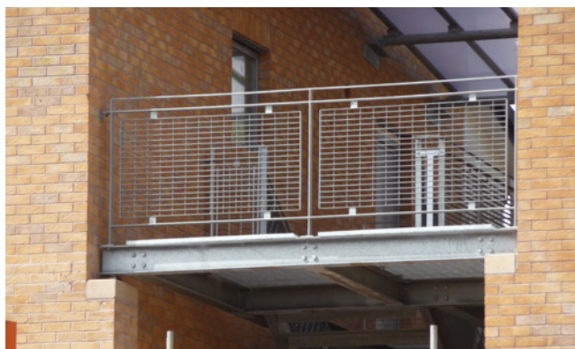
Figure 15 Robust, permanent staircases were installed in place of temporary access to speed up construction
