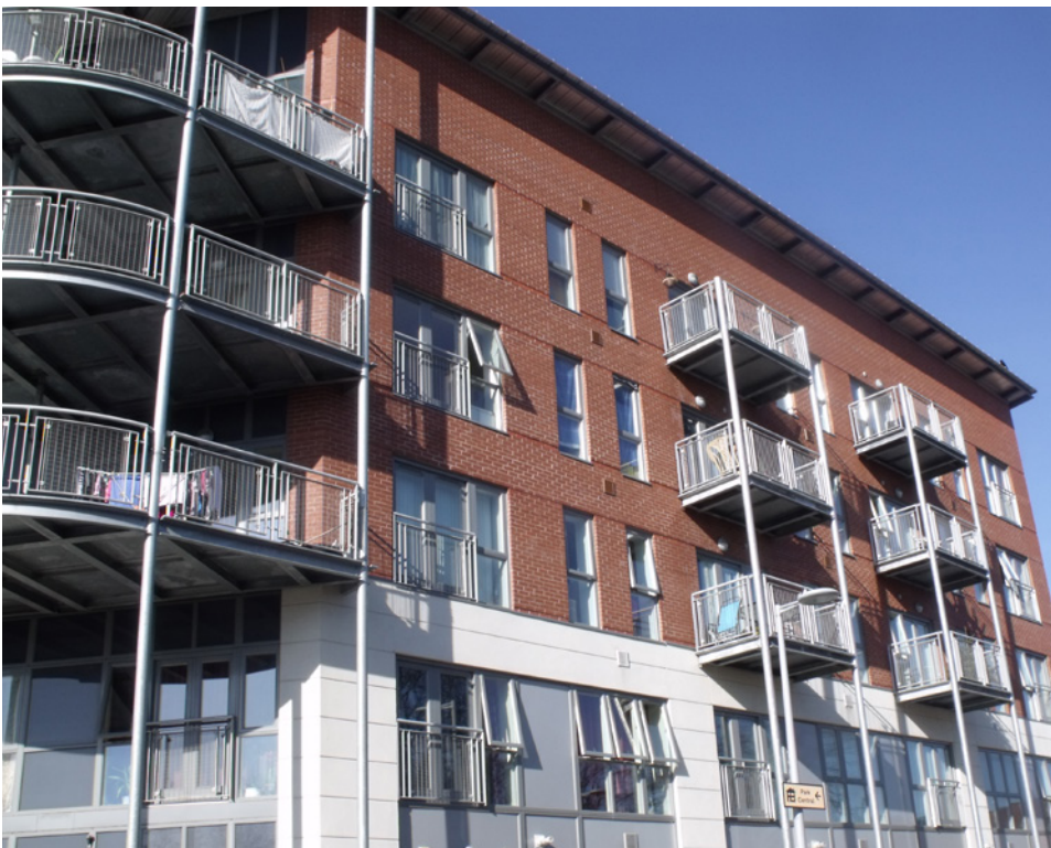
Figure 27 Block 78 at Park Central (Photo © Elliott Brown)
