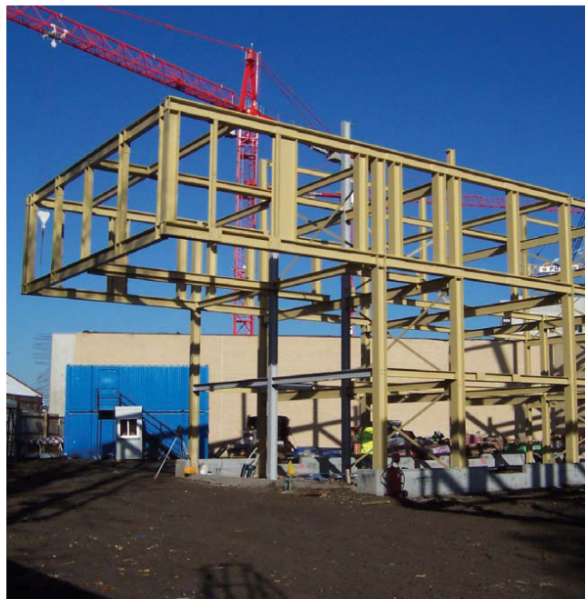
Figure 21 The cantilevered steel frame (© Tata Steel)
