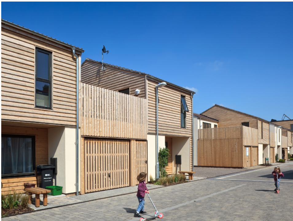
Figure 17 Terraced homes at Lime Tree Square (© Crest Nicholson)
