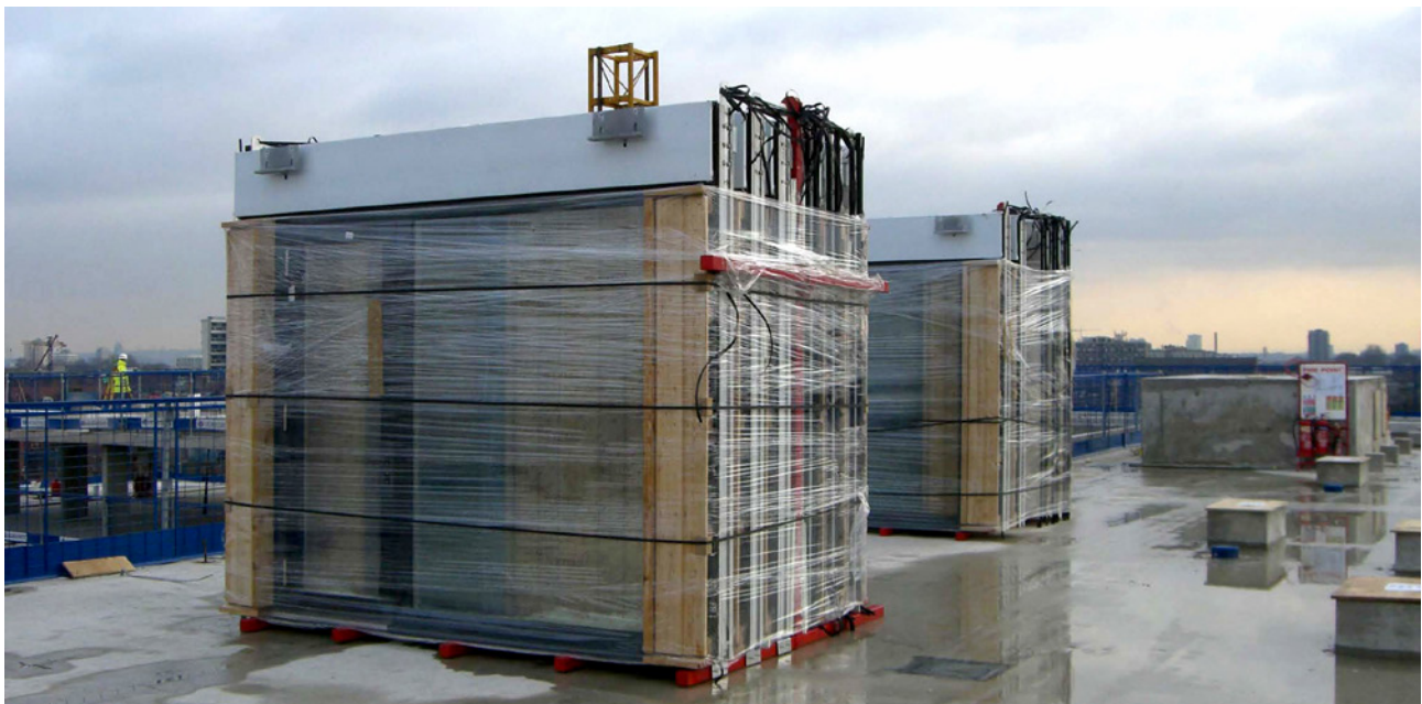
Figure 5 Packaged unitised cladding panels (© Allford Hall Monaghan Morris)
