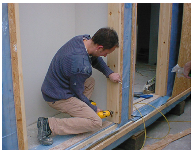
Figure 12 Timber framed panels were also constructed offsite
