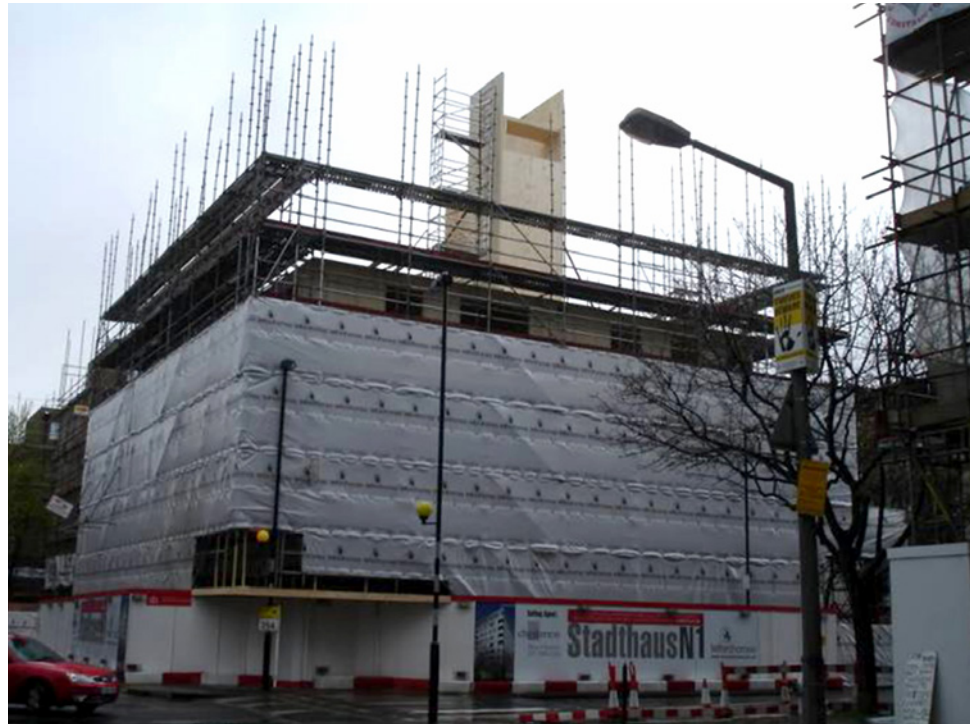
Figure 8 The Stadthaus under construction (© Waugh Thistleton Architects Ltd)
