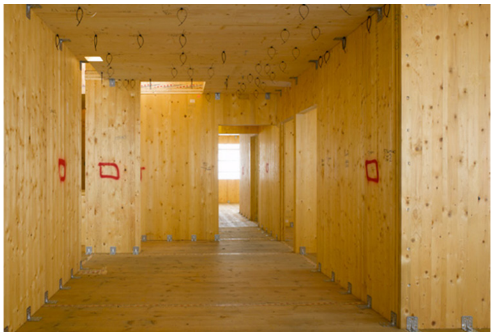
Figure 9 Exposed cross-laminated timber loadbearing walls and floors (© Waugh Thistleton Architects)
