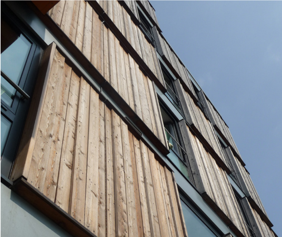
Figure 2 Unitised cladding panels
