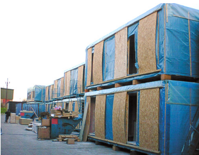
Figure 11 Volumetric units were constructed in Cambridgeshire before being transported to Leeds
