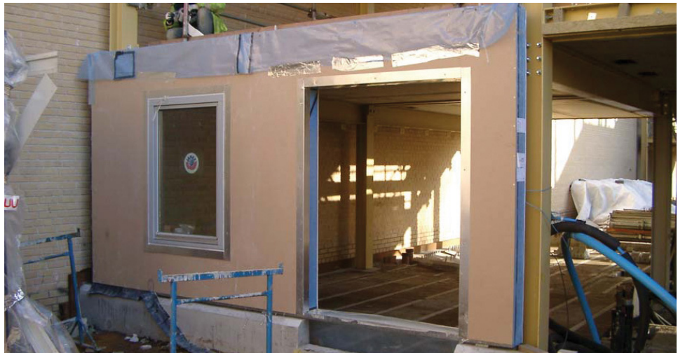
Figure 22 Wall panels arrived complete with windows (© Tata Steel)
