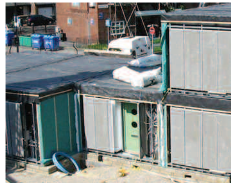
Figure 6 Weather protection on volumetric units.
