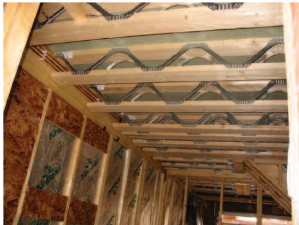
Figure 5 Metal web joists.
