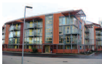
Figure 4 Solar shading – keeps out the midday sun but lets in the evening sun.
