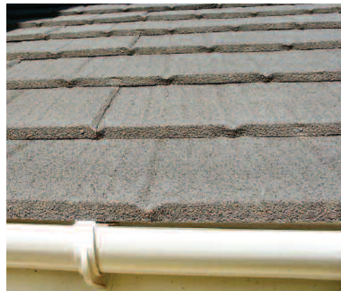
Figure 10 Modern lightweight roof covering made from profiled metal sheet.
