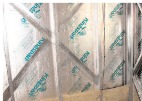
Figure 12 Bracing in light gauge steel frame construction.
