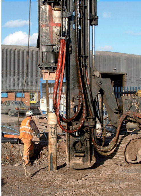
Figure 19 Installation of driven steel piles.
