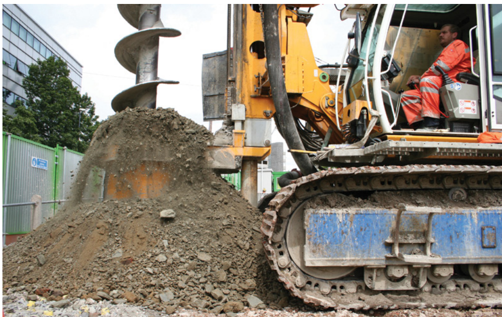
Figure 21 Continuous flight auger bored piling.
