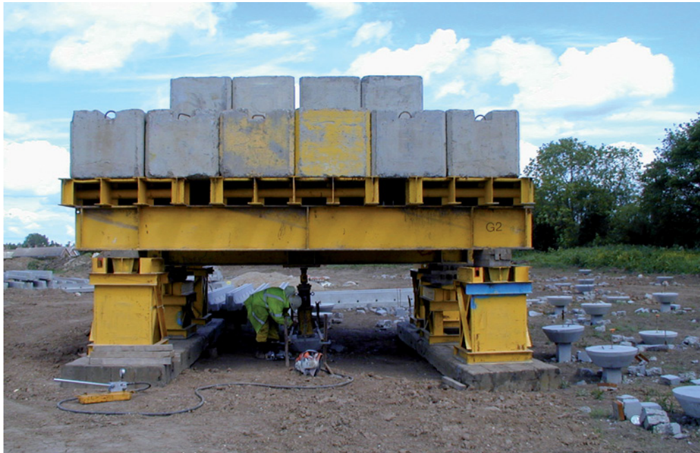
Figure 26 Static load testing of piles using kentledge.
