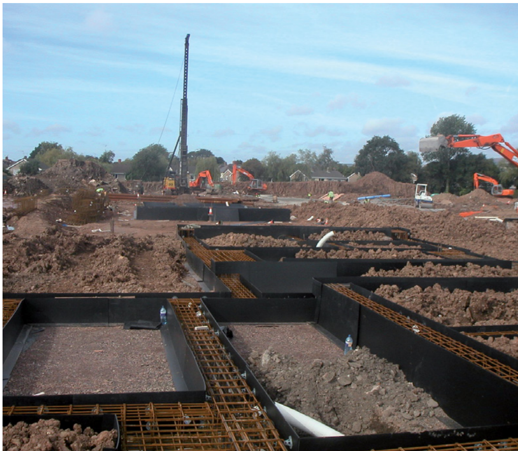
Figure 17 Ground beams prior to casting of concrete.
