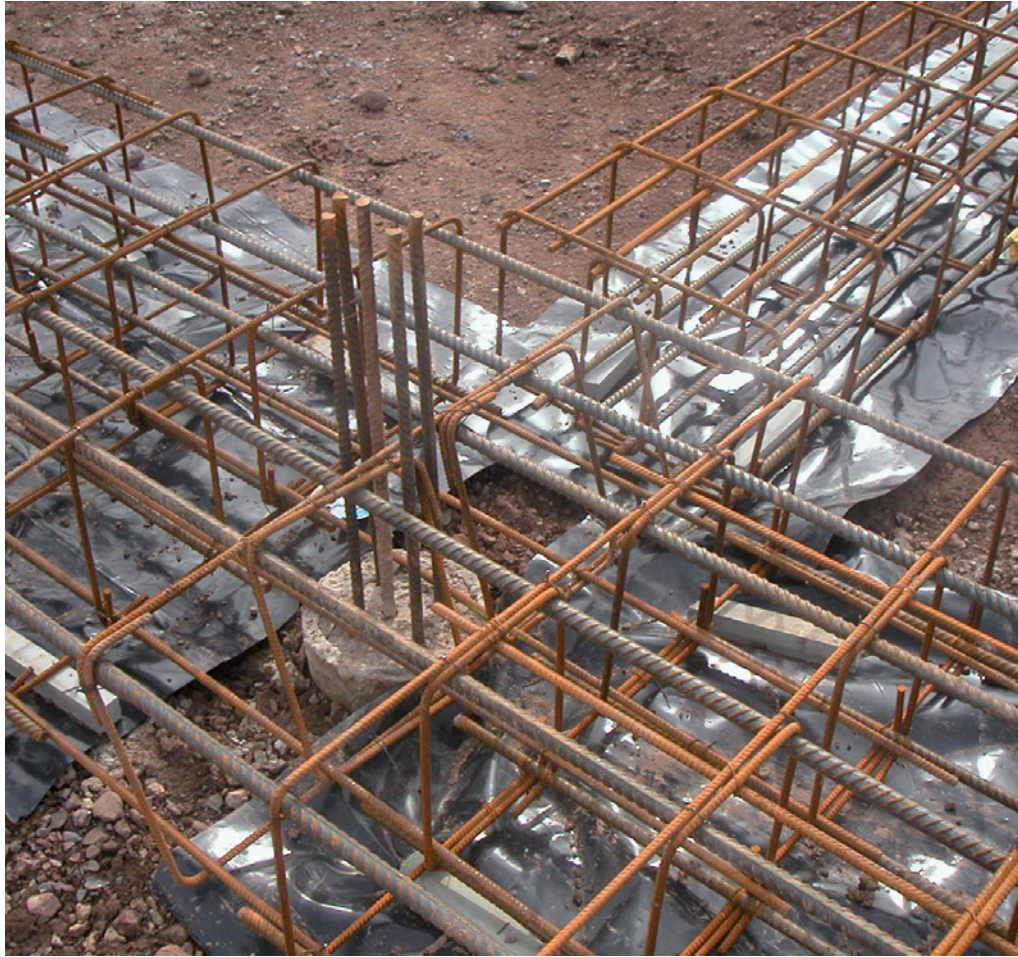
Figure 16 Pile and ground beam reinforcement.
