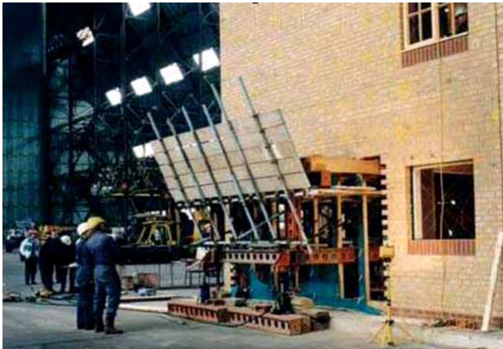
Figure 19 Disproportionate collapse test on TF2000 timber frame building
