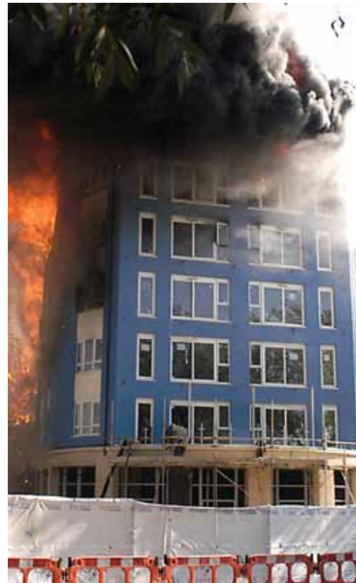
Figure 35 Fire spread to block B1 (reproduced by courtesy of the London Fire Brigade)
