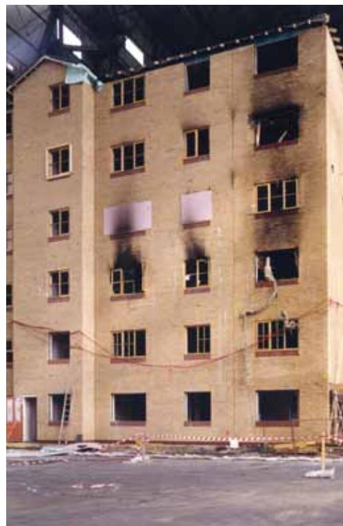
Figure 22 Front elevation of TF2000 building showing extent of vertical fire spread
