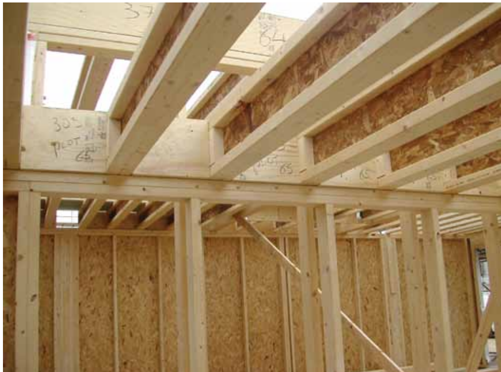
Figure 4 Engineered floor joists (photo courtesy of UK SIP Association)
