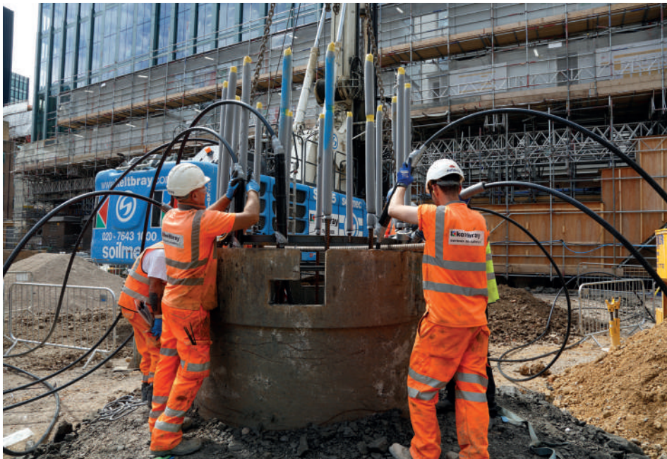
Image 13 Keltbray team installing traditional geothermal loops within solid piles (Source: Keltbray)
