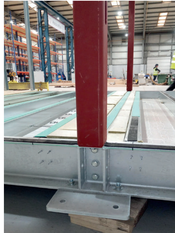
Image 12 Inbuilt ring beam foundation (Source: Elevate FBE Ltd.)
