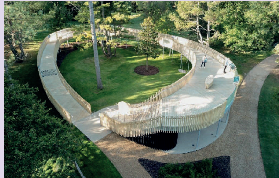
Image 11 RapidRoot installation along a public garden walkway (Source: RapidRoot)
