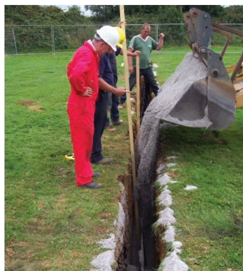
Figure 5 Installing horizontal ground loops
