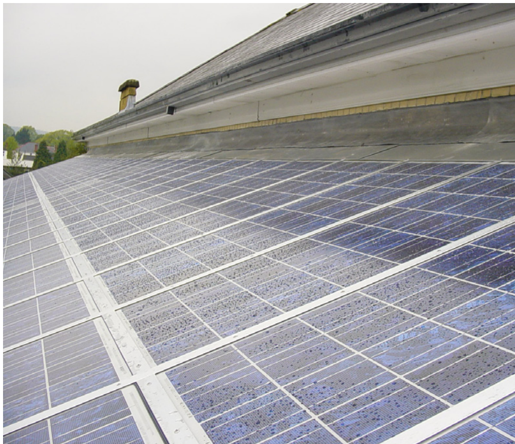
Figure 7 Integrated PV module system.
