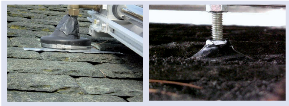
Figure 29 Examples of poorly sealed roof penetrations.
