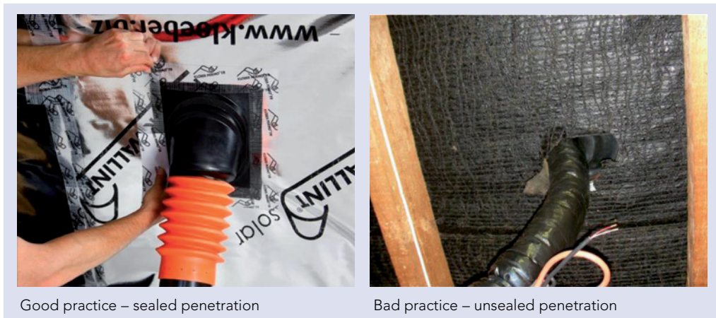
Figure 31 Examples of good and bad practice with underlay penetrations.
