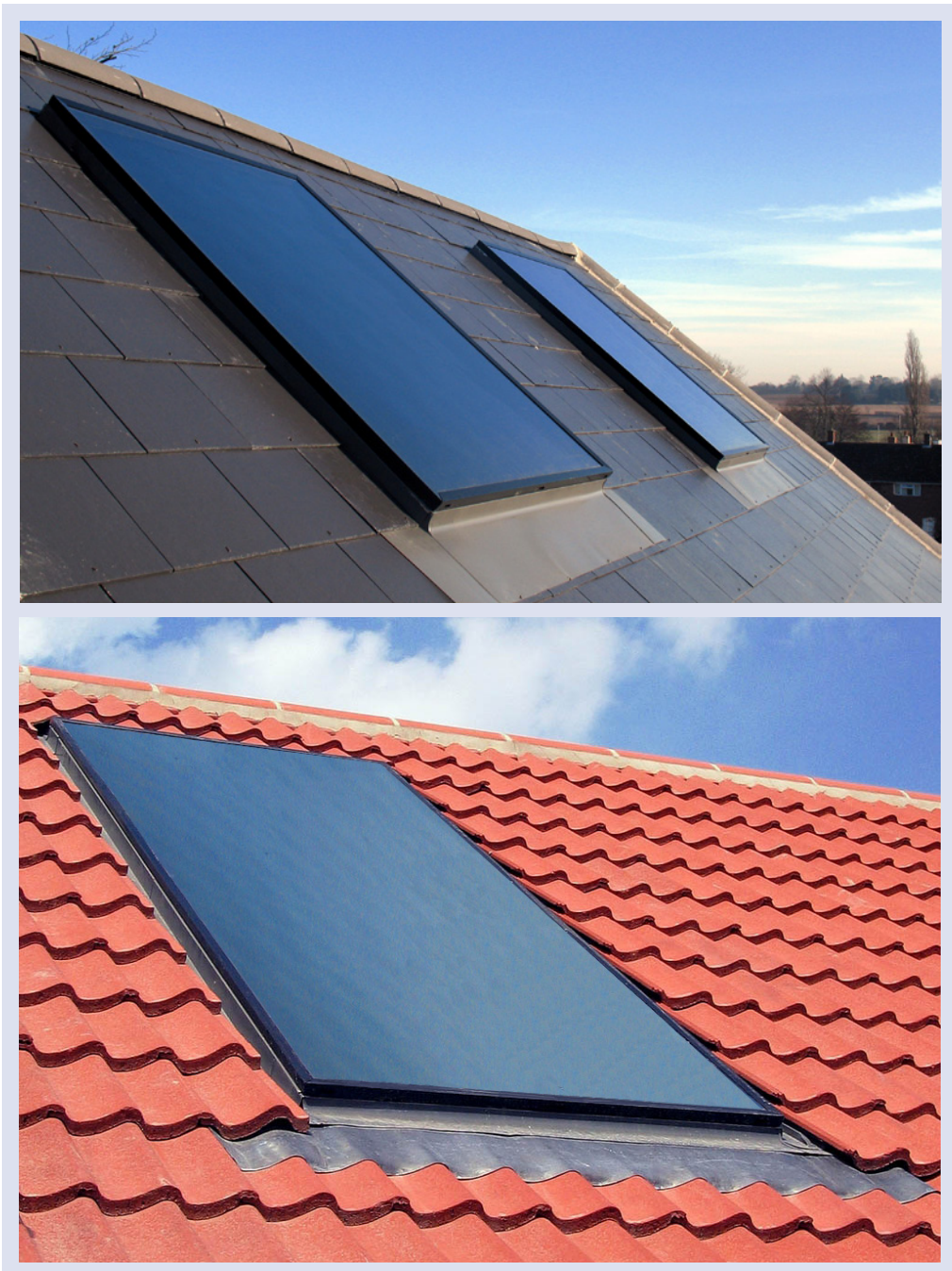
Figure 32 Integrated flat plate solar collectors with slates and profiled tiles.
