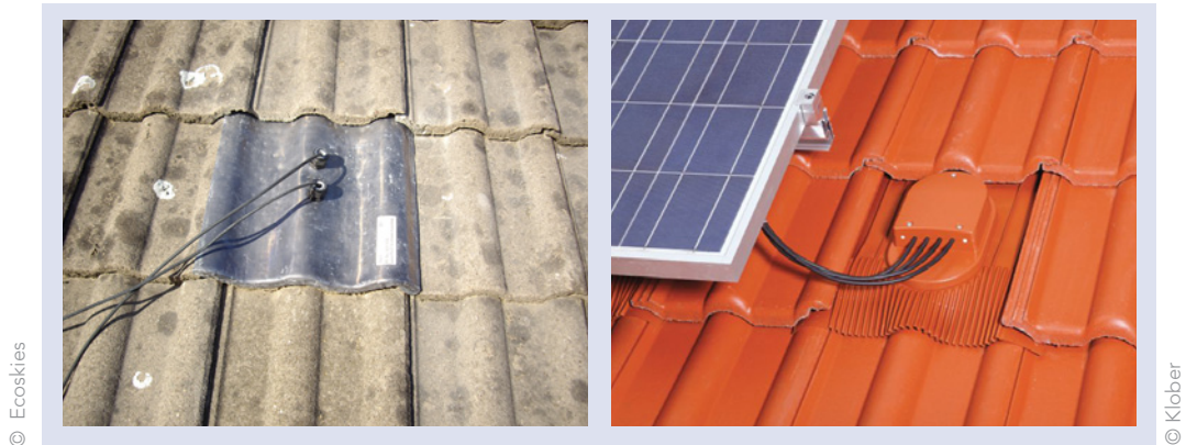
Figure 23 Purpose designed tiles to provide a weathertight entry for power cables.
