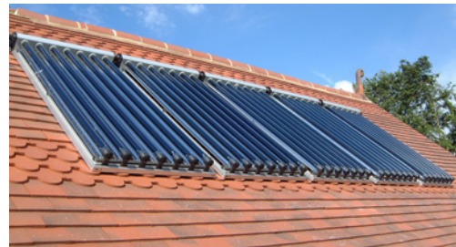
Figure 27 Evacuated tube solar collector.
