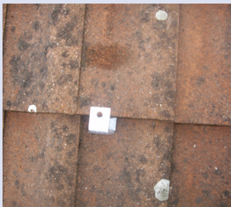
Hook fixing with tile in place
