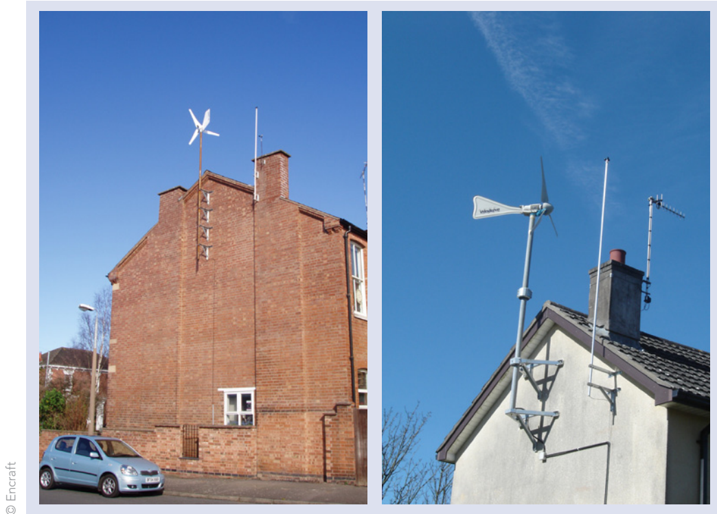
Figure 36 Typical microwind turbine wall fixing brackets.
