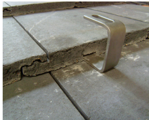
Figure 16 Single lap tile notched for hook fixing (note that the gap around the hook is similar to that between the tiles).
