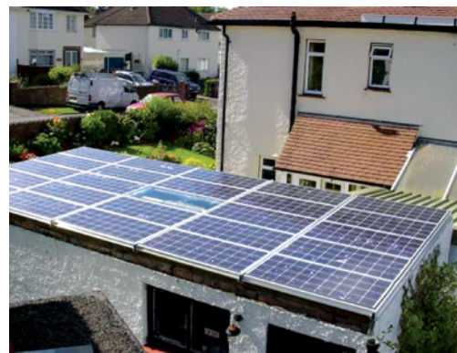
Figure 25 PV system integrated into a flat roof.
