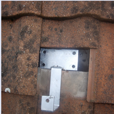
Single lap tile lifted to allow hook to be installed
