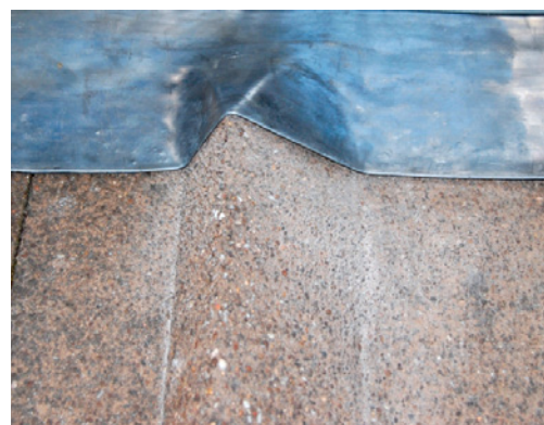
Figure 4 Flashing in place on trimmed tile.
