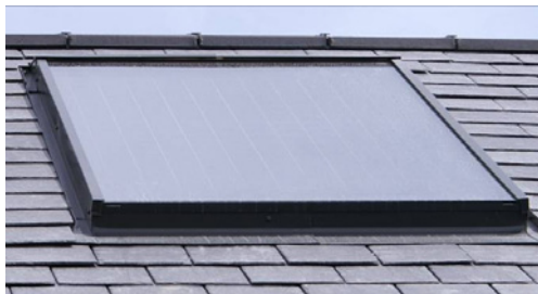
Figure 26 Flat plate solar collector.
