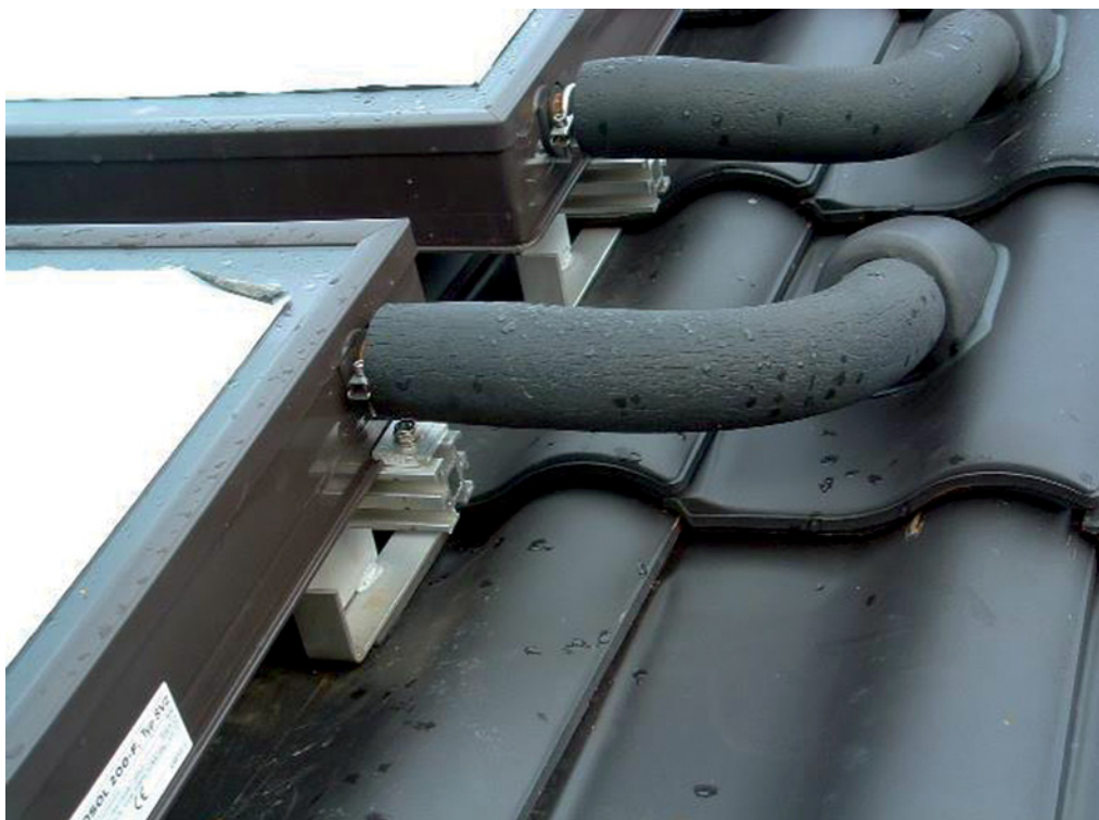
Figure 30 Example of weathertight penetration using a modified roof tile.
