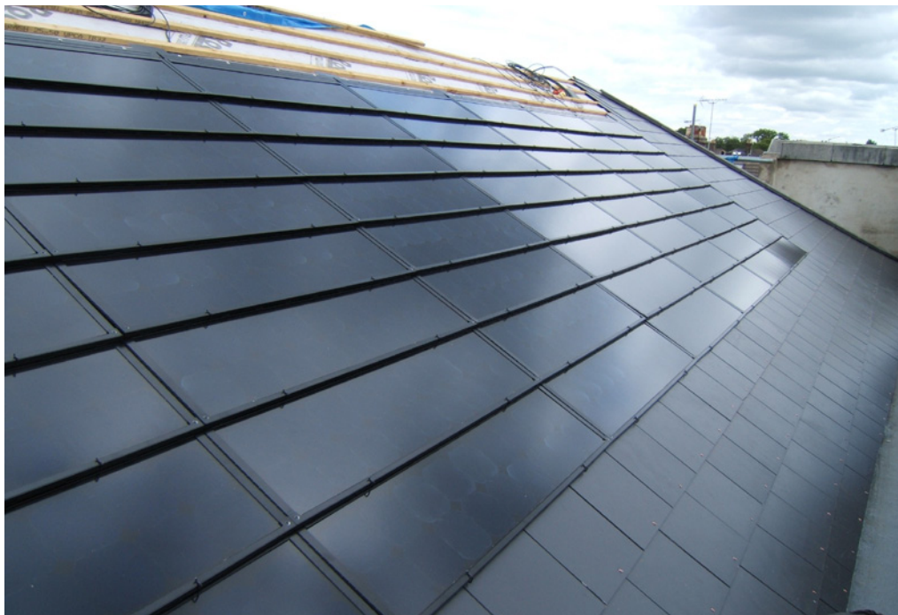
Figure 6 PV solar slate designed to interface with existing slates without additional flashing.
