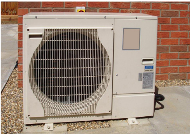
With ASHPs the main unit, which draws heat from the air, is located outdoors
