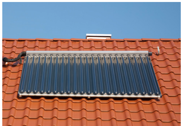
Solar thermal panel – usually one panel per house – may be tubular or flat
