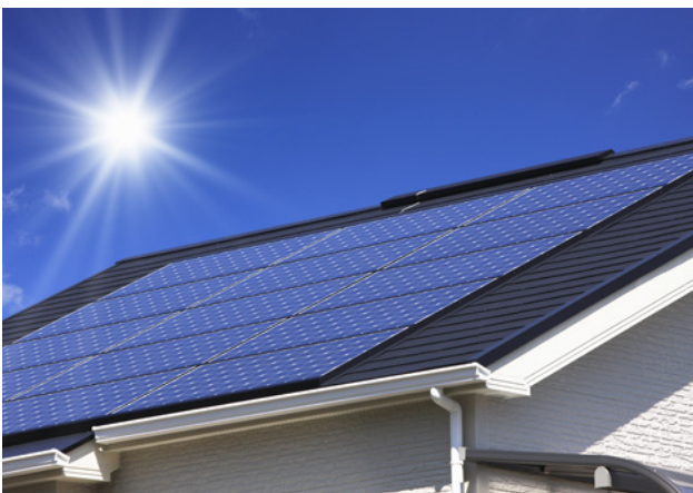
PV panels – often several flat panels per house. Panels (or sometimes PV 'tiles') may be integrated into the roof
