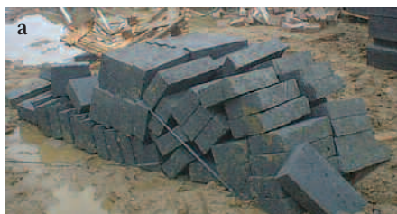
Figure 7a Poorly stored blocks become saturated with water in bad weather.
