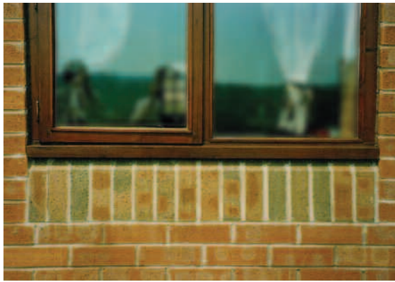
Figure 3a Flush brick-on-edge subsill.
