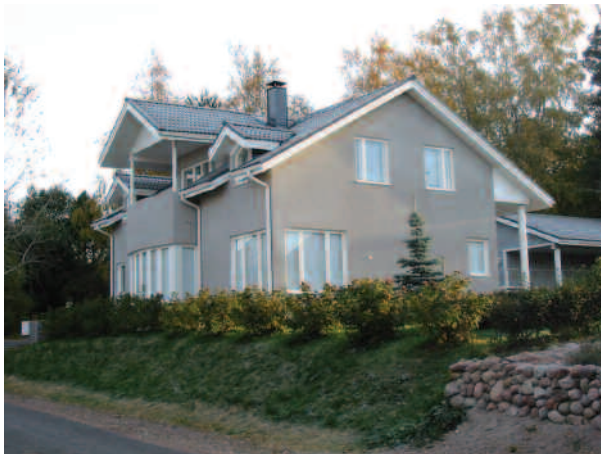
Figure 2 Generous overhangs at eaves and verge help to protect buildings from the weather.
