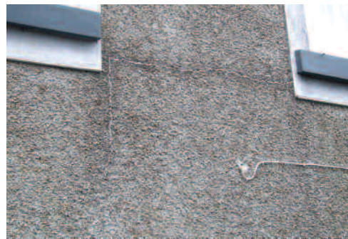
Figure 17 Repaired cracks in external render.
