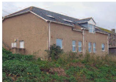
Figure 24 Careful detailing has given good performance in an exposed coastal location.
