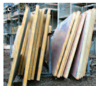
Figure 7c Timber framed panels awaiting installation. They are stored in a purpose-made frame and individually wrapped in polythene for protection.
