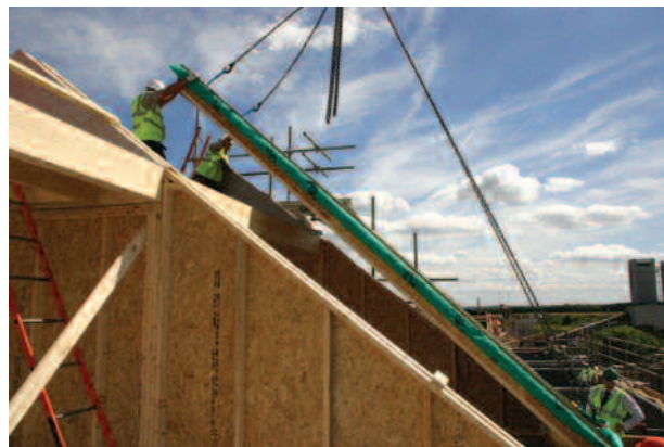
Figure 29 Roof cassettes being installed.
