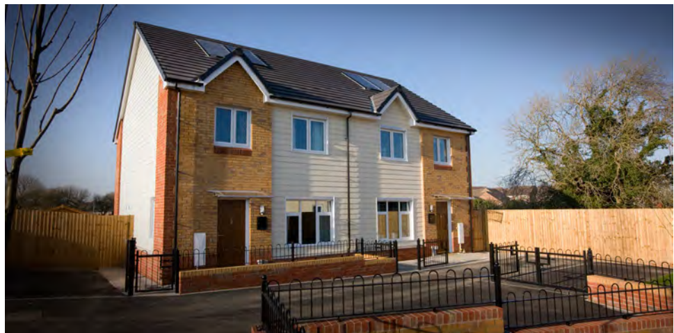
Figure 1 Traditional-style Passivhaus homes in Bridgend, Wales (© Hollbrook Homes Ltd)
