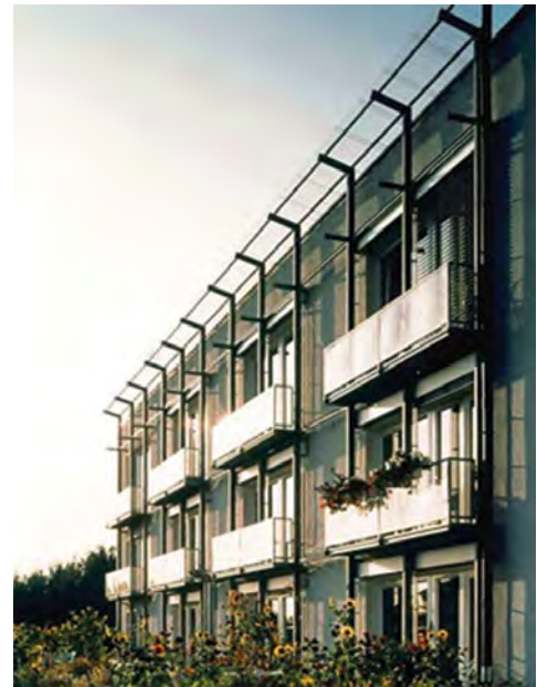
Figure 7 The first Passivhaus, built in 1991 in Darmstadt, Germany (© Passivhaus Institut/IPHA)
