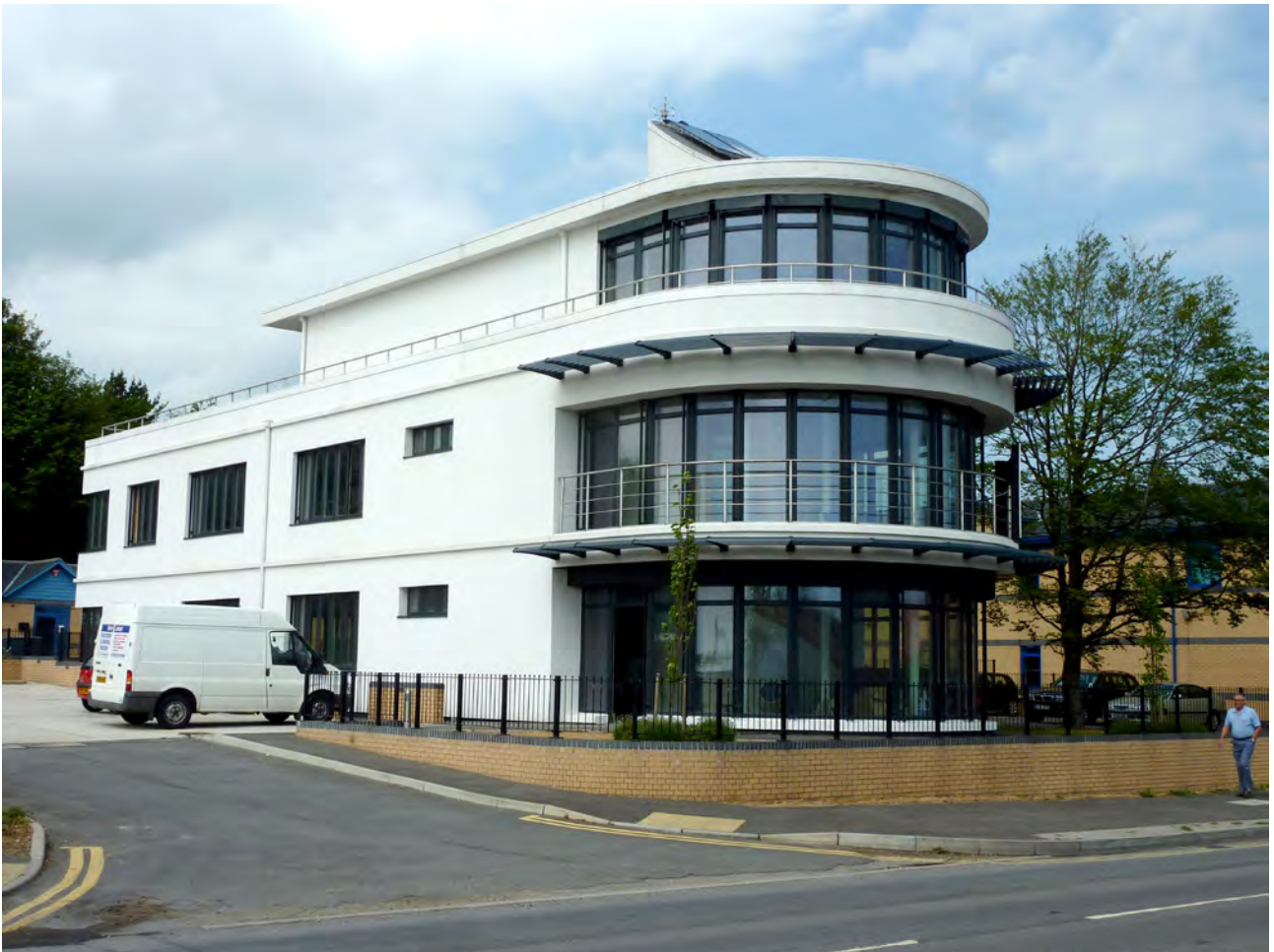
Figure 5 Passivhaus office in Dover, Kent (© Kym Mead, BRE/Dudley Marsh Architects)
