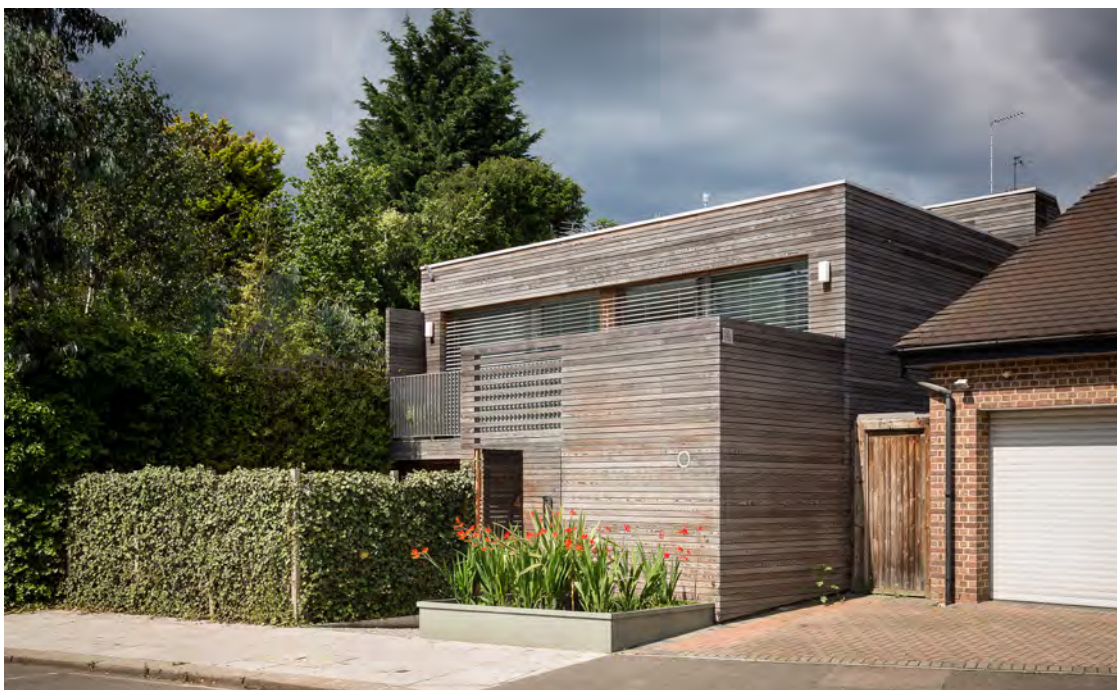
Figure 4 Contemporary Passivhaus home in Camden, London (© Tim Crocker)
