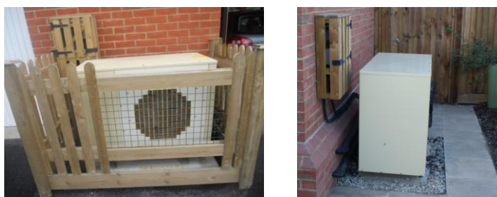
Figure A1 The ASHP unit with and without the fencing which smooths the airflow into the unit.
