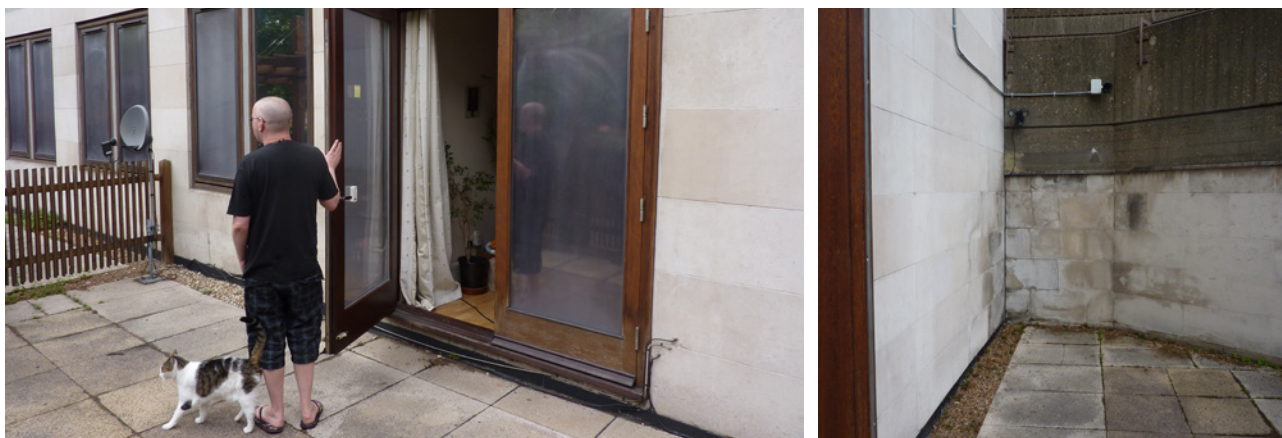
Figure 10 Bedroom window and patio doors looking onto paved garden area
