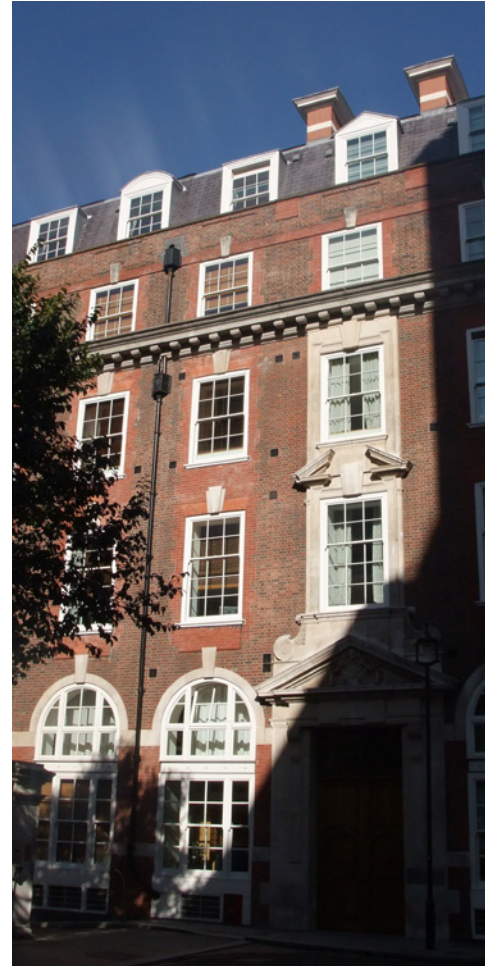
Figure 6 Flat within mansard roof
