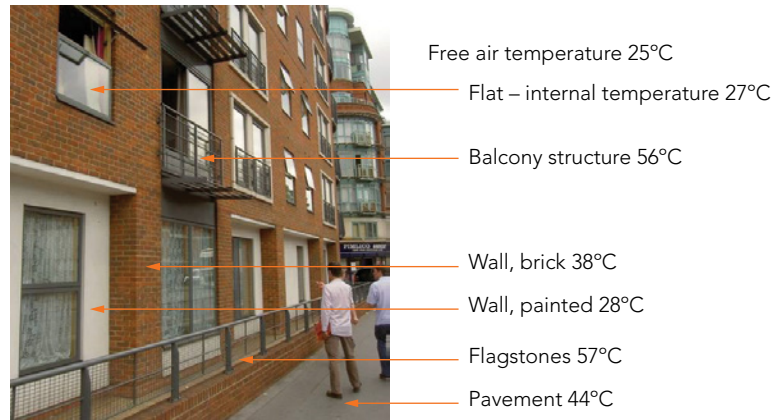
Figure 8 Air temperature and temperatures of building components and surroundings on a warm day
