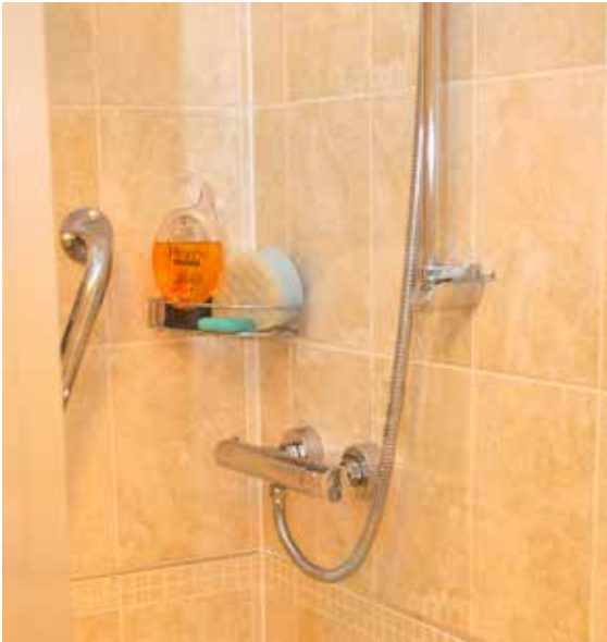
Figure 23 Shower controls were not always easy to operate due to lack of levers
