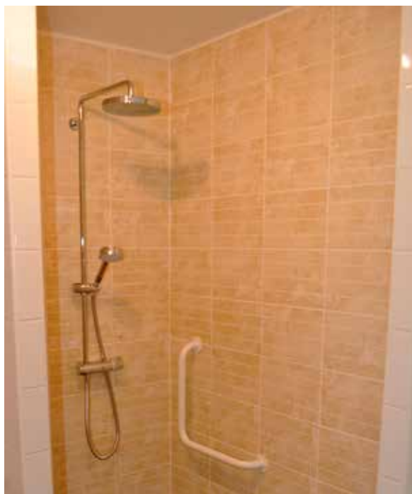
Figure 15 Grab rails were not always fitted in showers as standard
