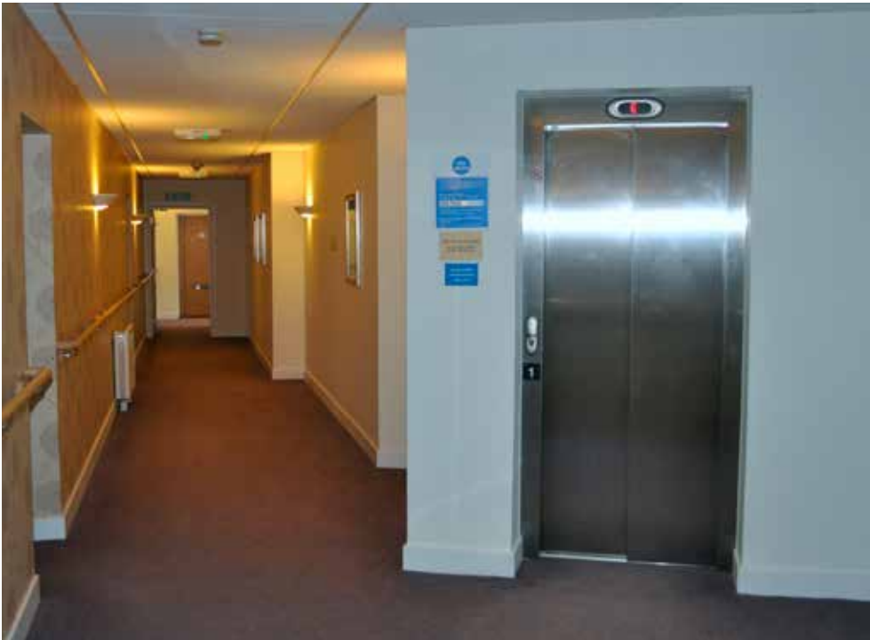
Figure 28 Lift with good access to upper floors and grab rails in corridors
