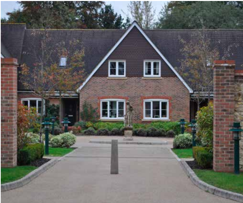
Figure 11 Communal space and outlook are important factors in choosing a retirement home
