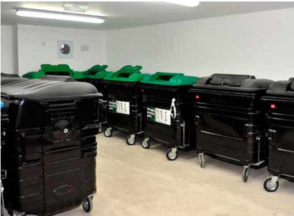
Figure 29 Refuse bins are all on one level with small easy access doors at the top for rubbish disposal
