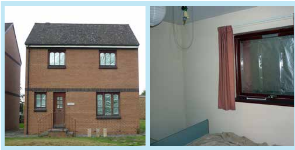
Figure 23 House B with aluminium foil directly attached to the glass on the inside of the window
