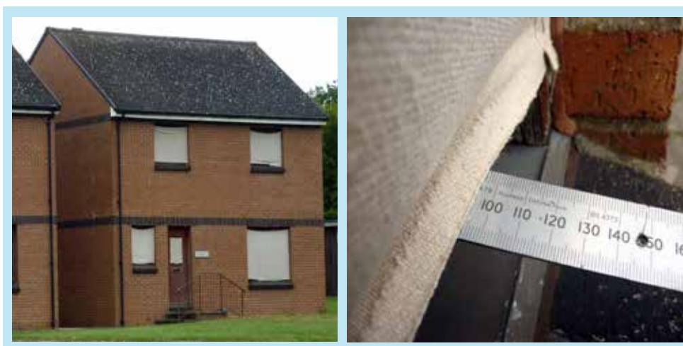
Figure 25 House B with heavyweight cotton fabric attached to the external wooden window frames (approximately 100 mm off the glass)
