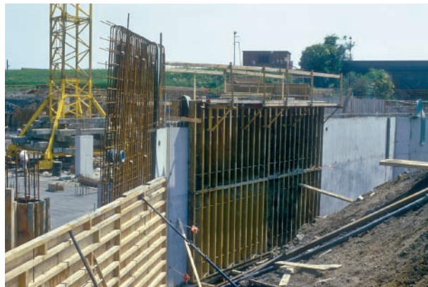
Figure 2 Cast-in-situ reinforced concrete.
