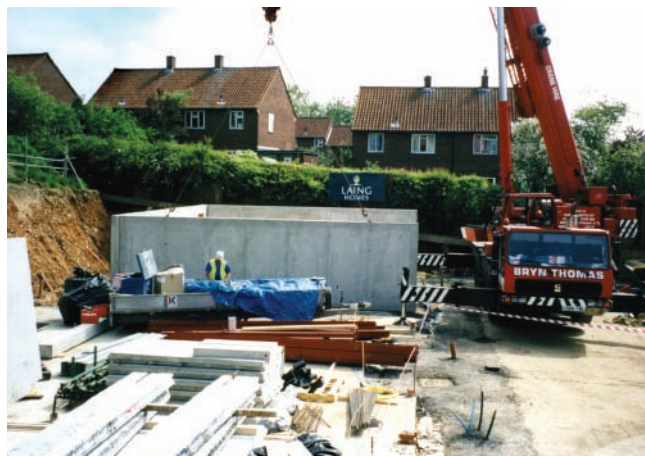
Figure 4 Precast insulated concrete panels.
