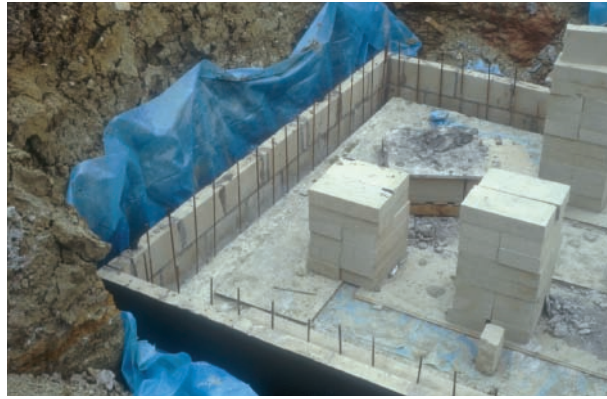
Figure 1 Blockwork walls (courtesy of The Basement Information Centre).
