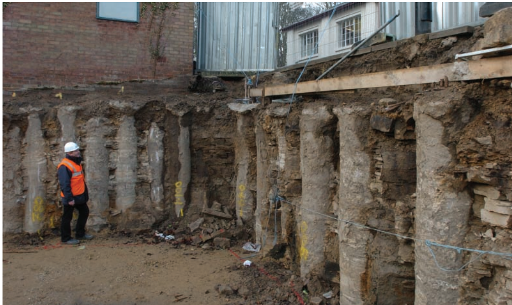
Figure 7 Contiguous piles after excavation.
