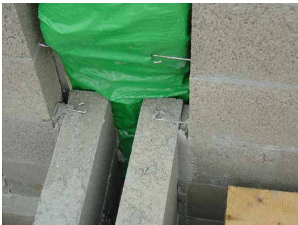
Figure 10 Minimising noise transmission (AD E E1) between new homes. The cavity sock provides fire protection and insulation against flanking sound transmission Photograph courtesy Robust Details Ltd
