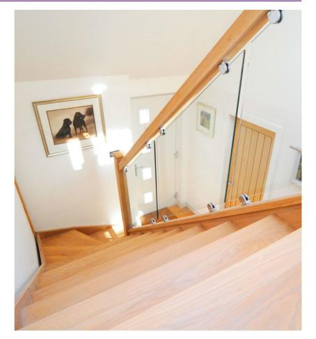
New homes are designed and built to modern Building Regulations requirements and have safety glass in areas where damage is possible or likely to cause an injury, for instance, in glass doors or low level windows.
