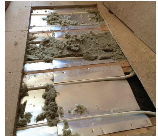
Figure 22 Insulation left over metal heat diffuser panels will compromise heat transfer and should be cleared prior to installation of floor finish
