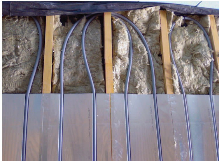
Figure 21 Mineral wool can also be used to insulate under diffuser plates in timber floors. The plates should be prevented from sagging so that thermal contact is maintained with the floor finish
