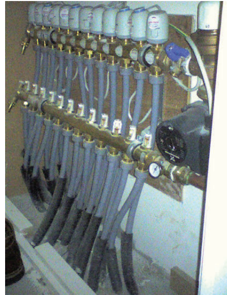
Figure 16 Insulation sleeves can be fitted over underfloor heating loops
