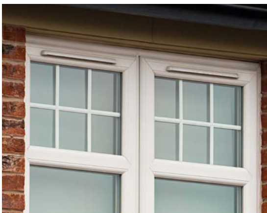
Figure 8 Trickle vents incorporated in a casement window
