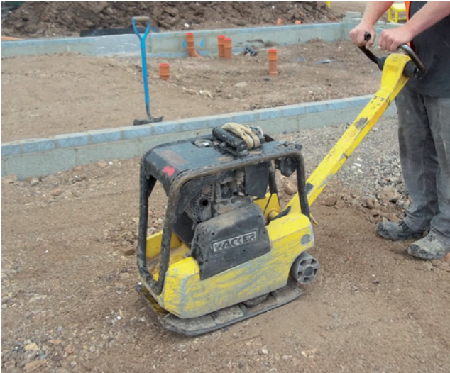
Figure 2 Hardcore being compacted (© Bellway Homes East Midlands)
